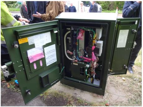
Twelve fibres were installed on the aerial route alongside the copper phone cable, connecting to a new box in the village with Huawei's termination equipment (left). Just one fibre is lit for broadband, and as this is shared between just 70 homes rather than the usual 200 to 300 there will not be a problem with contention. This also leaves the village well placed for the next generation G.fast rollout of speeds of 400 to 500Mbit/s in 2016 and 2017.
